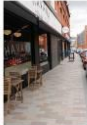
High quality natural stone paving to footways – enhancement of streetscape and opportunity to re-integrate 'old' culture
